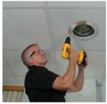
2- DRILL HOLES WHERE MARKED AND INSERT ANCHORS PROVIDED.
