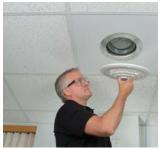
4— CENTER GRILL ON INSTALLED METAL RING TO ENGAGE MAGNETS AND ADJUST AS NEEDED TO COVER RING.
