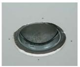
1- USE GALVANIZED METAL RING TO POSITION AND MARK **SCREW HOLES ON CEILING.**
